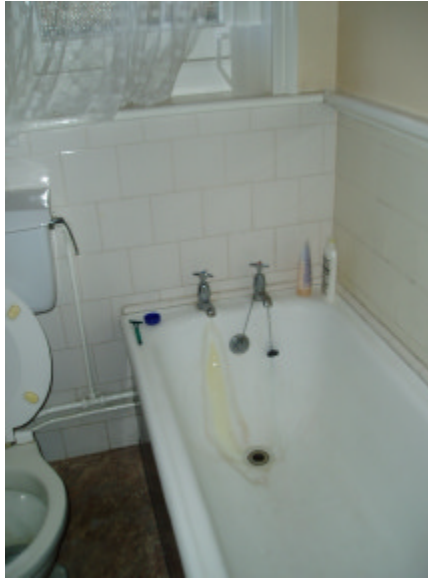
Figure 9 - A 67 Glisson Road Bathroom
