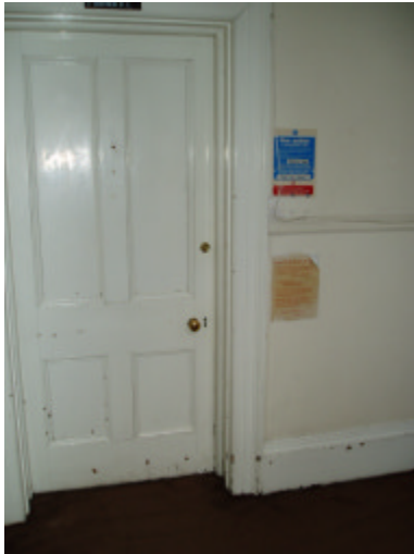
Figure 5 - Chipped paintwork
